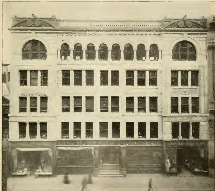
Central Exchange Building.
